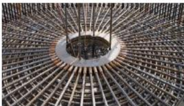
Figure 14: Lower zone reinforcement.
