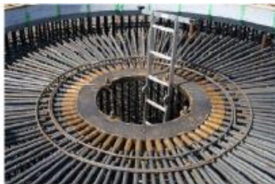
Figure 15: Upper zone reinforcement.
