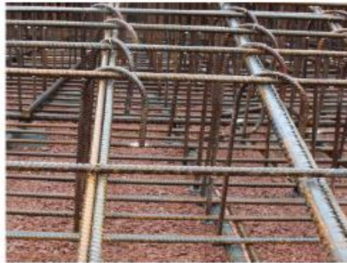
Figure 16: Web reinforcement.
